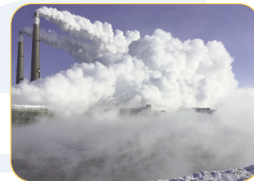
>>> Coal Creek Station Power plant during the Polar Vortex – Full Steam Ahead
